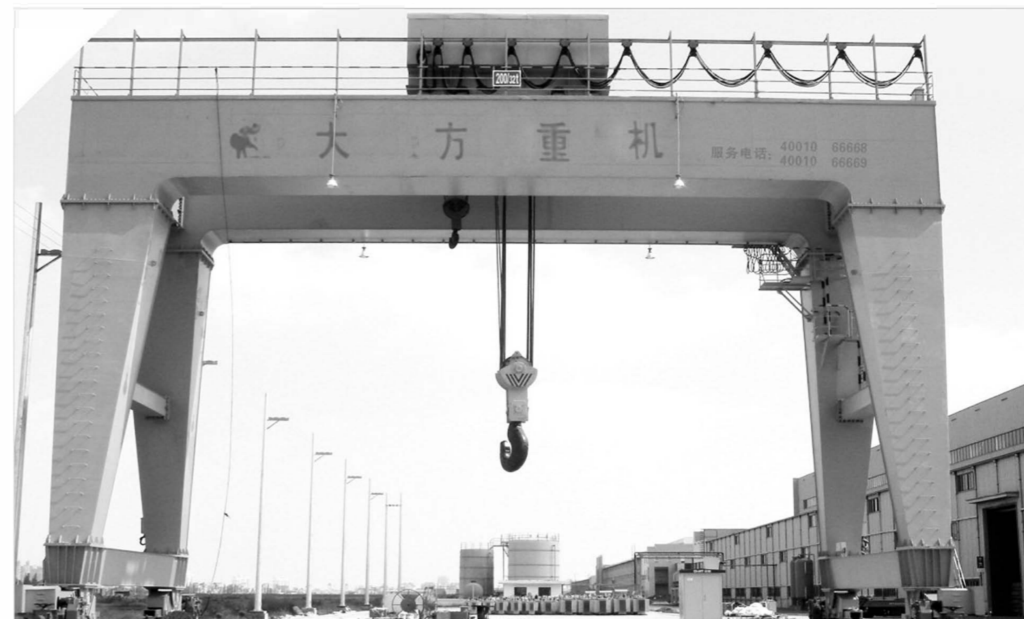
大方重机 卓越服务 MACHINERY AND EQUIPMENT
