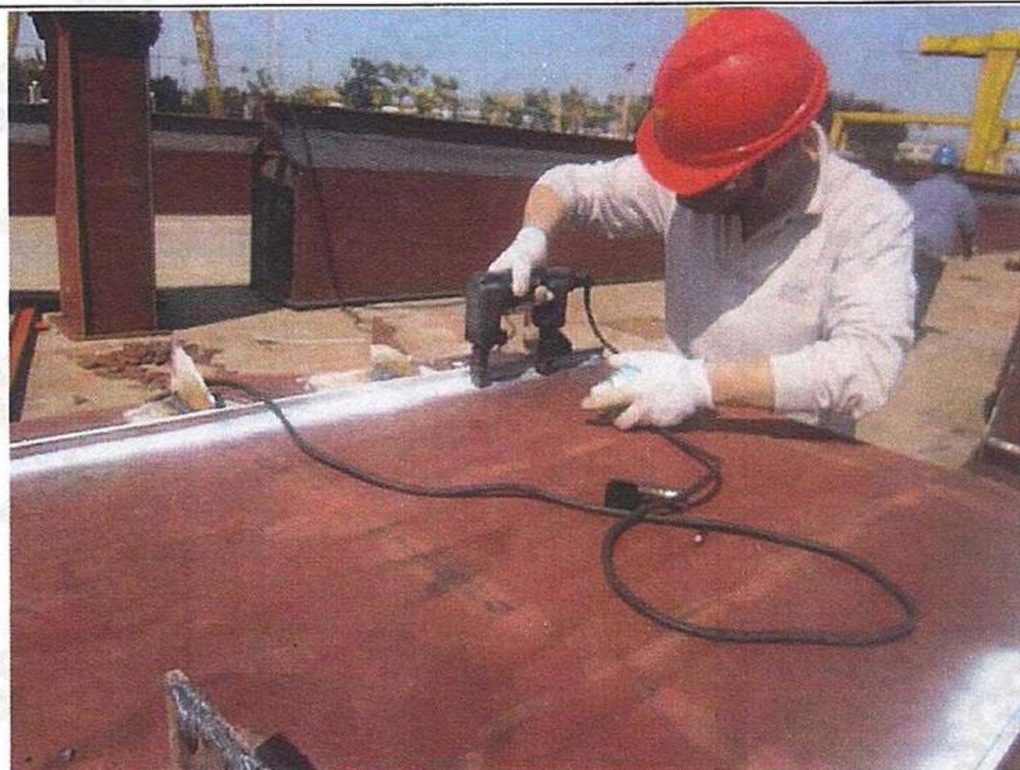
Photo5 MT for fillet weld
